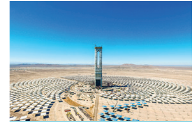
Solar Tower Receivers & Steam Generators
