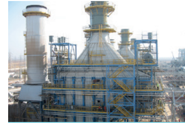
Heat Recovery Steam Generators
